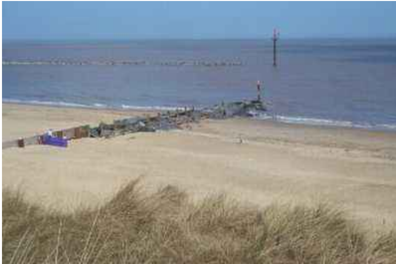
Rock reinforced original wooden groynes near Sea Palling, Norfolk at the termination point of the offshore rock reef, seen out to sea.
