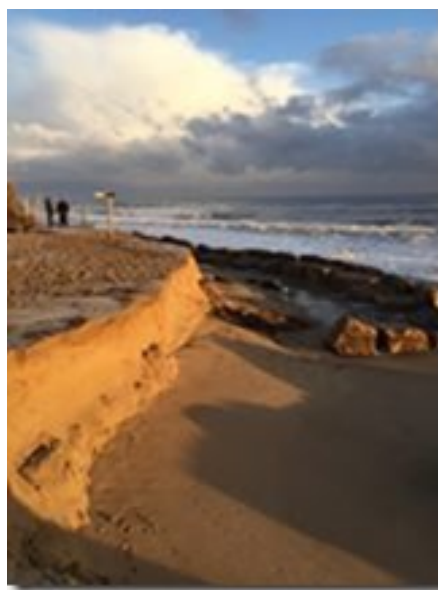
Erosion of beach and the natural sea defence system at Hemsby, Norfolk, following a tidal surge.
