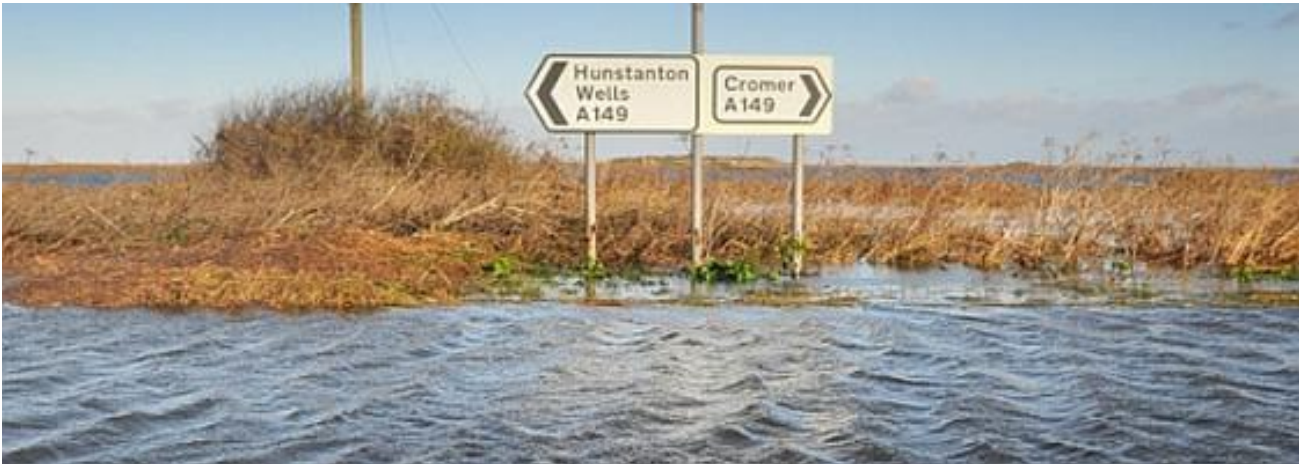
Norfolk main coast road following a tidal surge.
